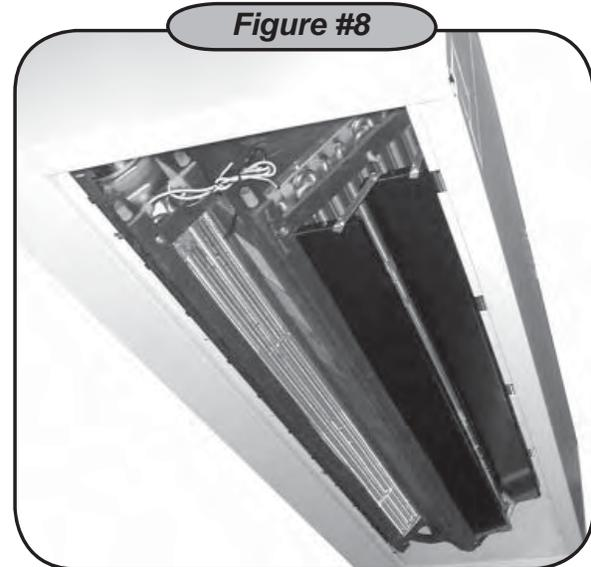
Drain pan extension installation complete – Ceiling configuration shown.
