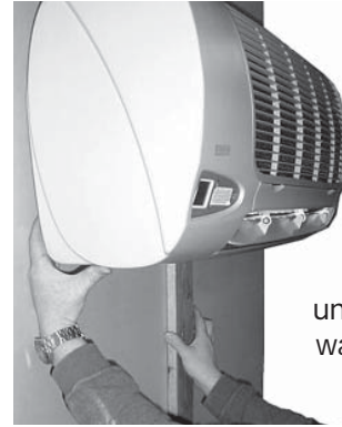
Figure 15 - Removing End Cap
