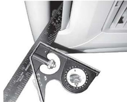
Figure 22 - Adjust Louver Position 30° From Plumb
