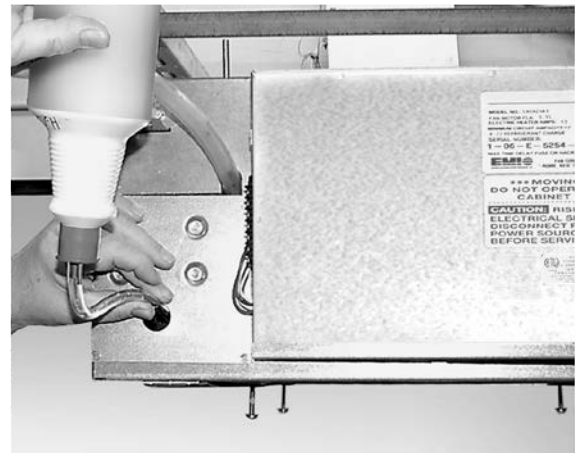
Figure 34 - Check Condensate Pump Operation
