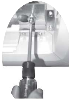
Figure 22 - Adjust Louver Position 30° From Plumb
