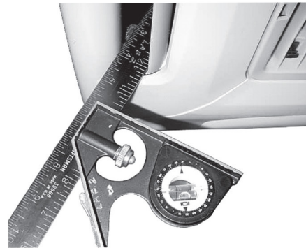
Figure 22 - Adjust Louver Position 30° From Plumb
