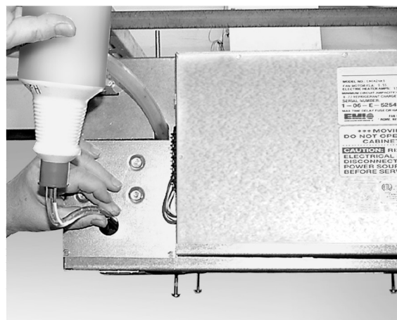
Figure 34 - Check Condensate Pump Operation
