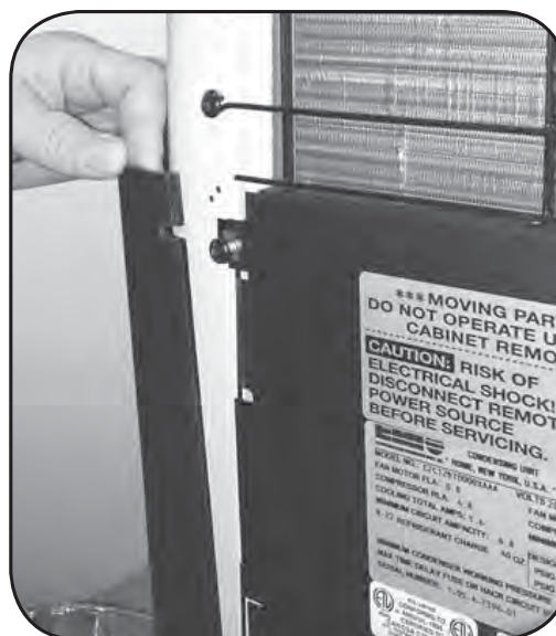
Figure 12 Replacing side panel
