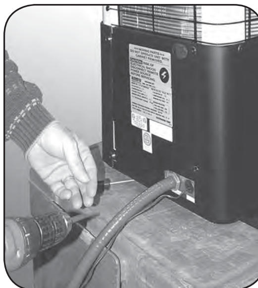
Figure 13 Fasten loose screws
