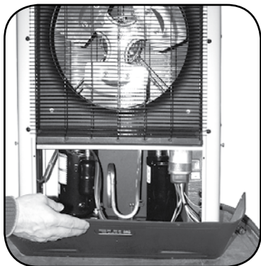
Figure 2 Remove front panel
