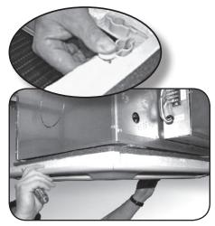
3. Lift the fascia onto the chassis mounting bolts. Align the key hole brackets with the mounting bolts and slide the fascia forward to lock into position.
