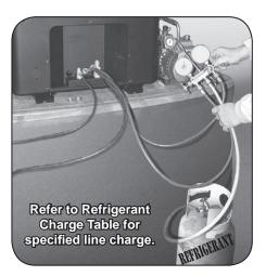
8. Charge to proper weight, charge based on the length of interconnect (see below).
