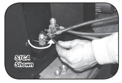
Once certain of a good evacuation and leak free joints, back-seat the valves (counter-clockwise) to open and allow factory charge to fill lines and indoor unit.
