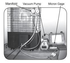
Evacuate line to 500 microns or less to ensure all moisture has been removed and there are no leaks.
