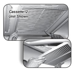
2. Remove the filter by carefully twisting and lifting to clear the retaining clips.
