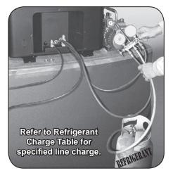
Charge to proper weight, charge based on the length of interconnect (see below).
