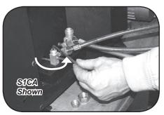
Once certain of a good evacuation and leak free joints, back-seat the valves (counter-clockwise) to open and allow factory charge to fill lines and indoor unit.
