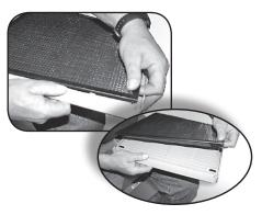
Lift the filter off the grille. Place filter on a flat surface and vacuum any away dust and debris (vacuum all filters and grills), also vacuum any accessible parts on the unit.
